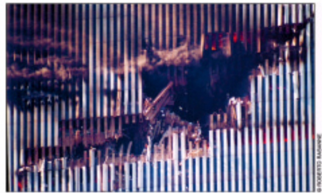
Figure 2-13 Impact damage to the north face of WTC 1.
