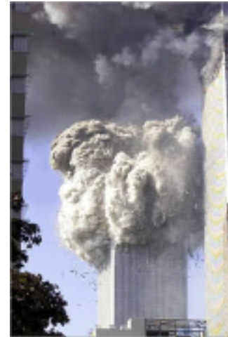
Figure 8: Progressive Collapse (Source: Internet - unknown)
